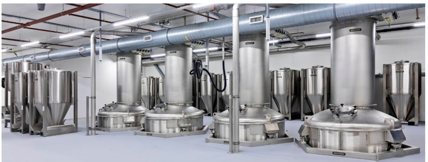
10.000 l weighing bins above the high performance mixing lines.
